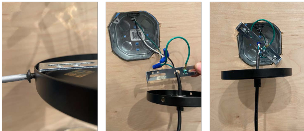
Fig.2a: Separate mounting bracket from canopy by removing set screws.
